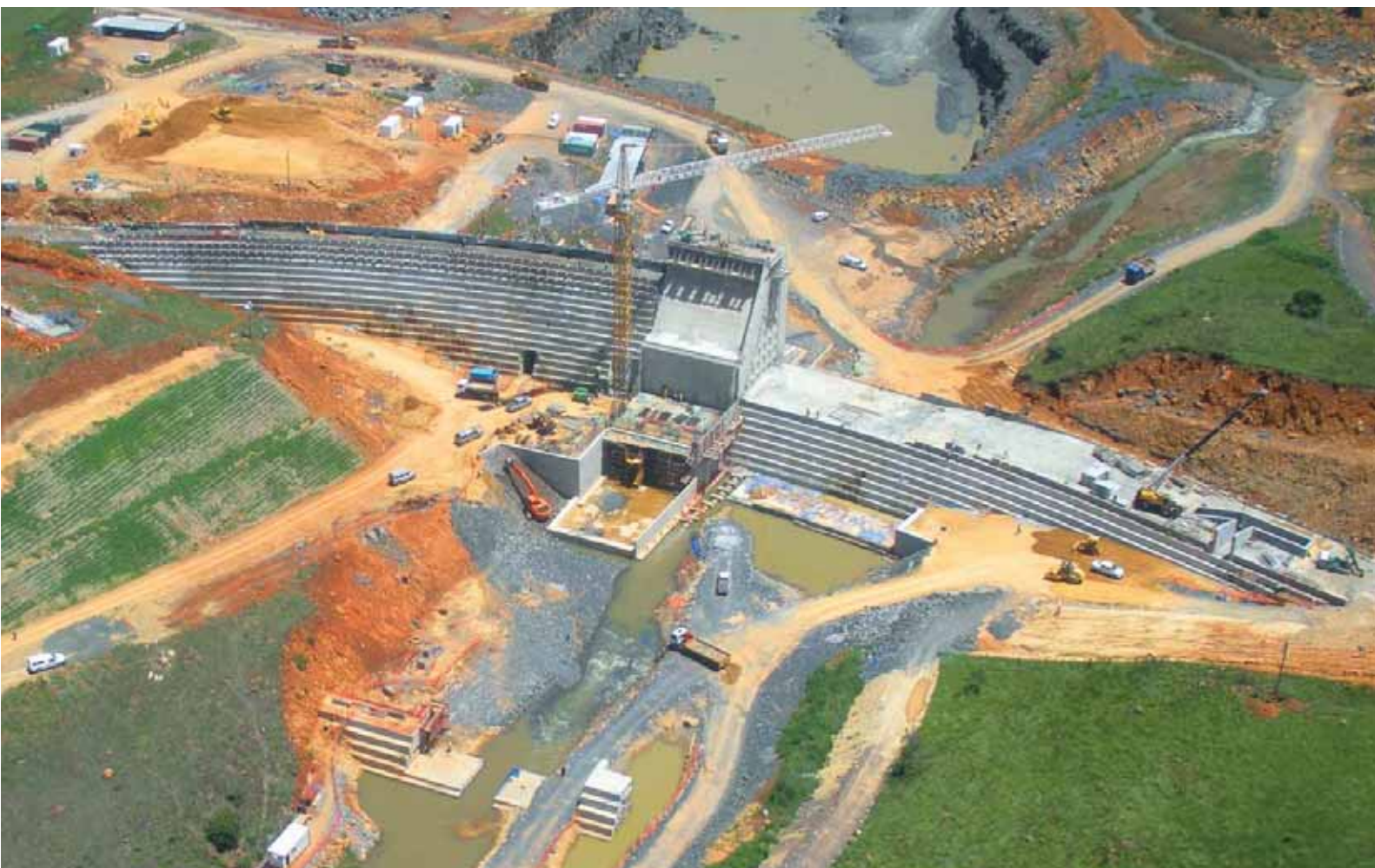
Bramhoek and Bedford Dams
