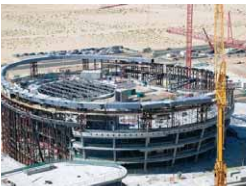
Zayed University library under construction
