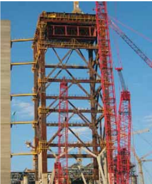
Heavy lift at Medupi
