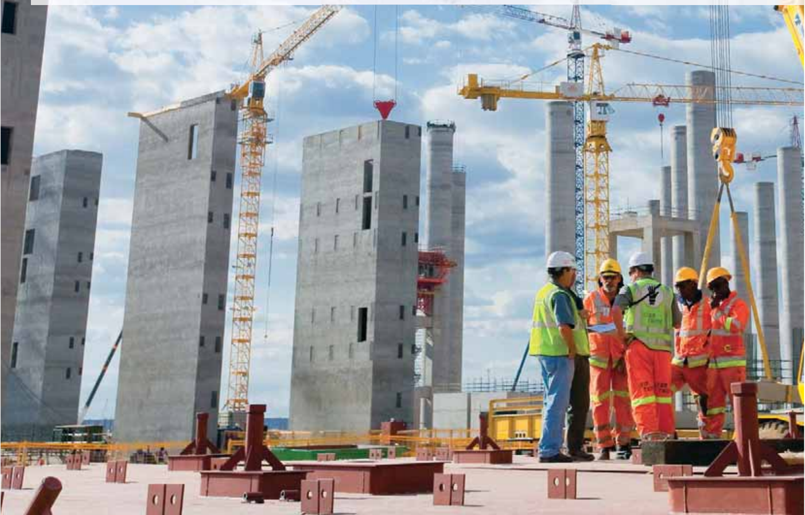
Medupi power station construction site
