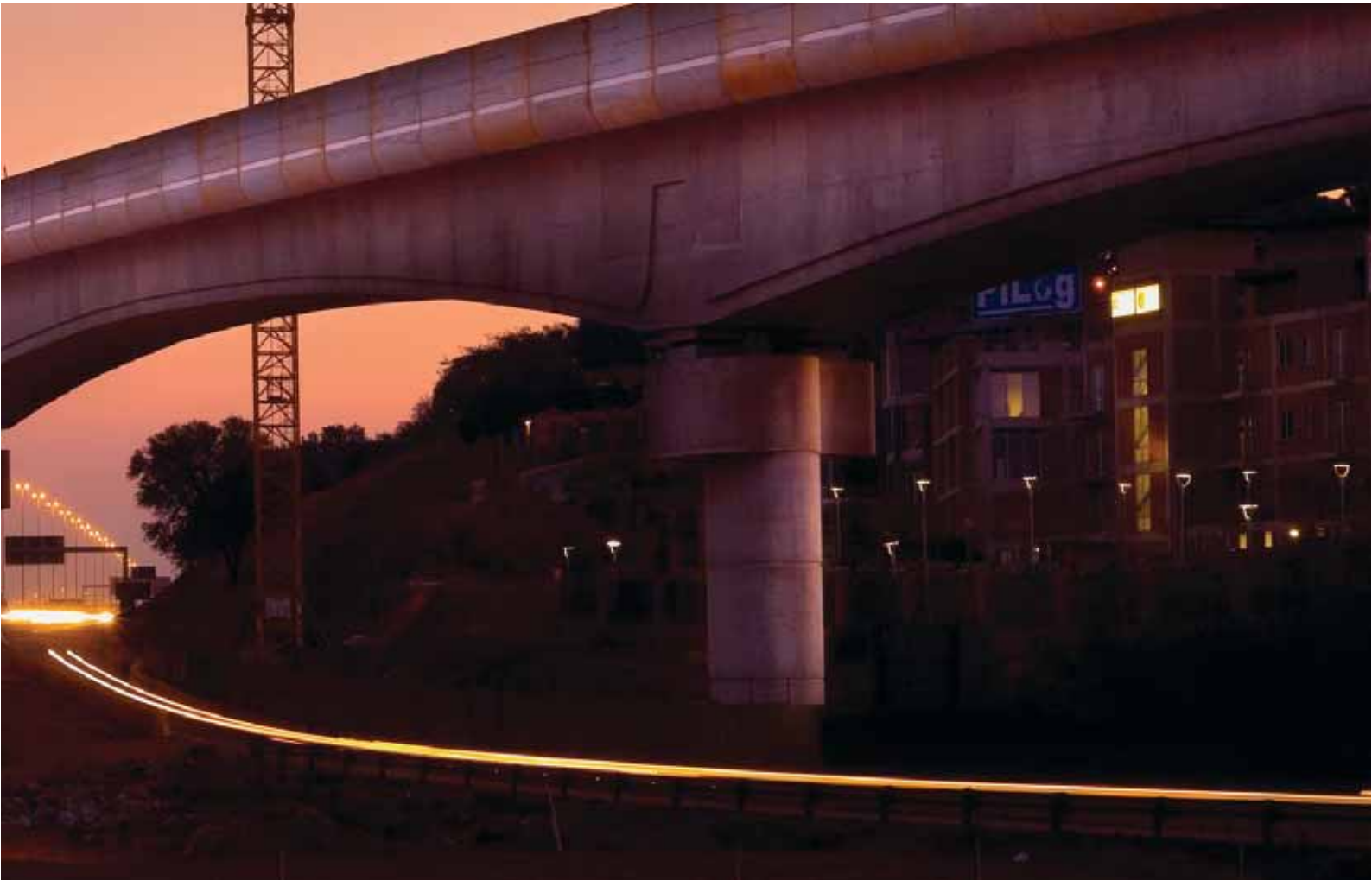
Gautrain viaduct under construction at Centurion, Tshwane
