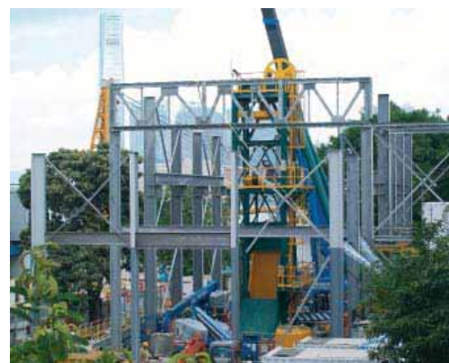
Wan Chai sewerage works, Hong Kong
