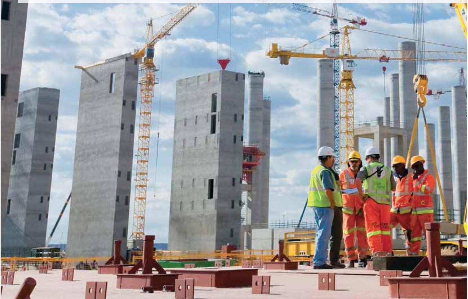
Medupi power station construction site
