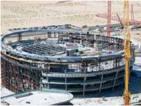
Zayed University library under construction
