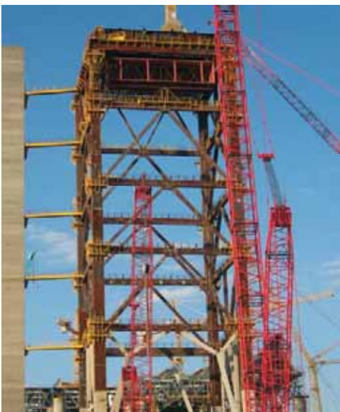
Heavy lift at Medupi
