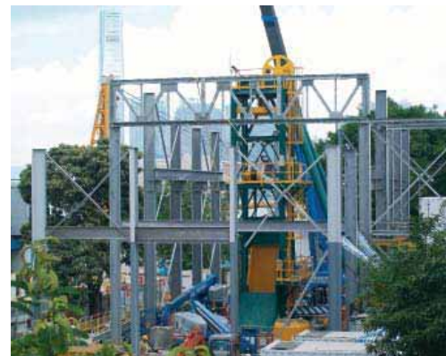
Wan Chai sewerage works, Hong Kong
