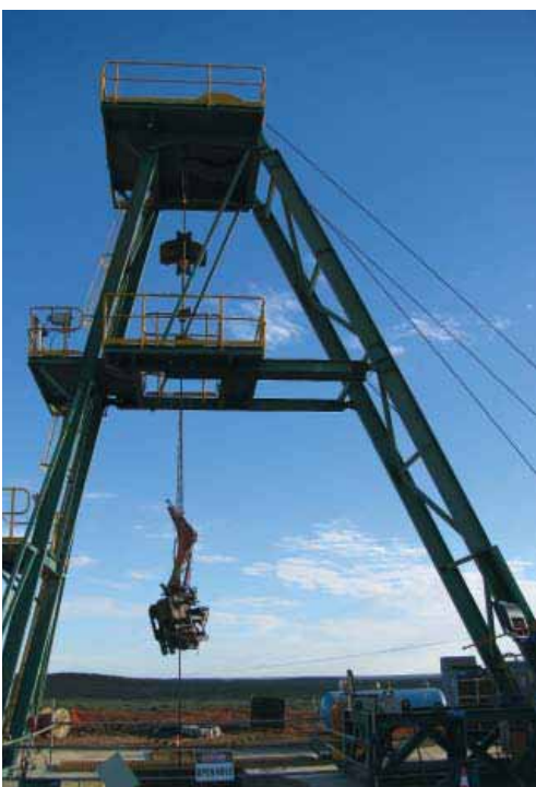
Gossan Hill shaft head during slinging operation
