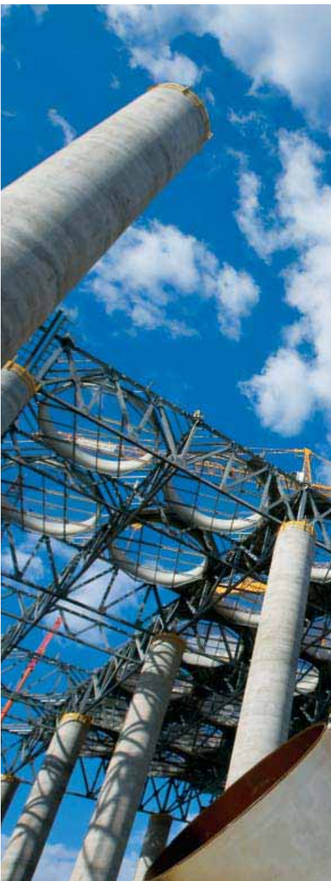
Medupi power station air cooled condensers
