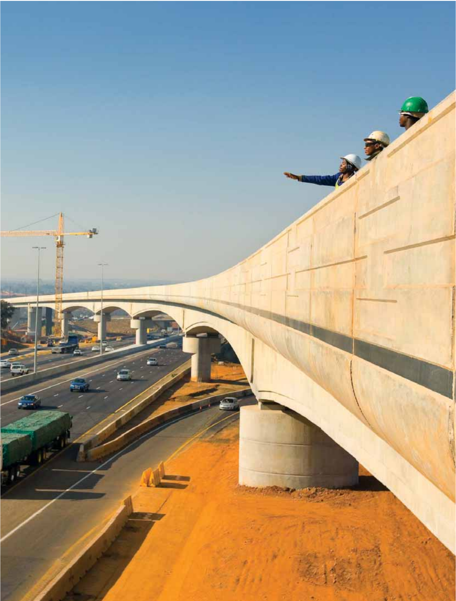
Gautrain viaduct at Centurion, Tshwane
